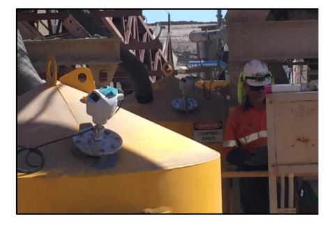
The radar level transmitters were installed and aligned without the plant being ready to run. Upon plant start up, it was found that the rock shelves within the hoppers were causing major process related issues, introducing problems that no level transmitter could overcome, mainly, product stacking up in the bin and resulting in only 20% of volume being live load.
