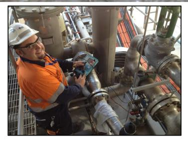
Instrowest Technicians worked hard to ensure the deadline was met. All instrumentation was tested to full scale at 25% increments and the findings recorded on our electronic calibration sheets.
