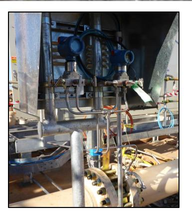
Instrowest Technicians found several issues during our calibration and commissioning work that also had to be rectified. These included instruments with incorrect ranges, incorrect wiring, and unattainable 1:20 fall on tube work requiring Instrowest to engineer a solution, all of which were rectified.
