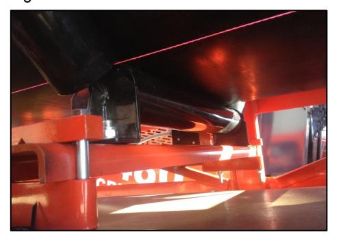
Instrowest worked alongside an OPS boilermaker to fabricate the custom brackets required to mount the belt scale and cut out the fixed trough idler between stringers. By utilizing the onsite boilermaker, Instrowest was able to reduce the installation cost and duration.
