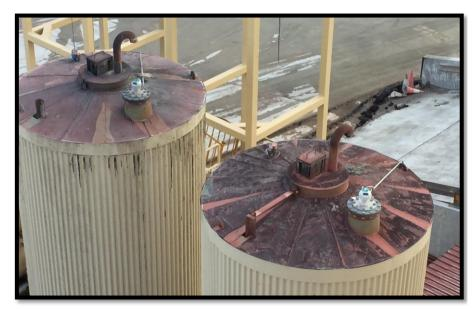
Fig 1: The two Siemens LR200's as installed on top of the Bitumen tanks.
