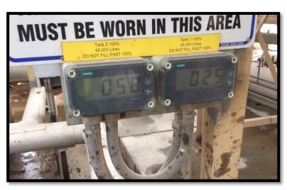
Fig 3: Two Siemens RD200 Remote Display's in their own IP68 enclosures mounted at ground level for field operators and the truck driver loading the tanks.
