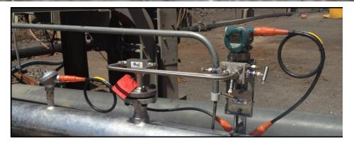
Once the capital was approved, Instrowest set about ordering the equipment which consisted of two Yokogawa Verabar flow elements (averaging pitot tubes) with EJX110A DP transmitters, a Yokogawa EJX530A Gauge Pressure Transmitter for system pressure and two PT100 RTD's and thermo wells with Yokogawa YTA70 "Puck" style temperature transmitters.
