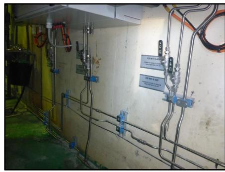
Figure 1: Analyser Tubing
