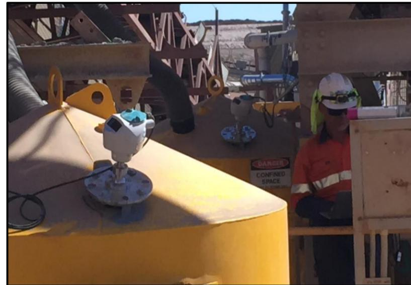
The radar level transmitters were installed and aligned without the plant being ready to run. Upon plant start up, it was found that the rock shelves within the hoppers were causing major process related issues, introducing problems that no level transmitter could overcome, mainly, product stacking up in the bin and resulting in only 20% of volume being live load.
