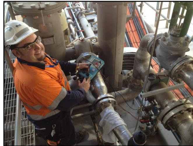
Instrowest Technicians worked hard to ensure the deadline was met. All instrumentation was tested to full scale at 25% increments and the findings recorded on our electronic calibration sheets.
