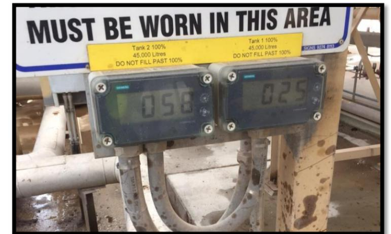
Fig 3: Two Siemens RD200 Remote Display's in their own IP68 enclosures mounted at ground level for field operators and the truck driver loading the tanks.
