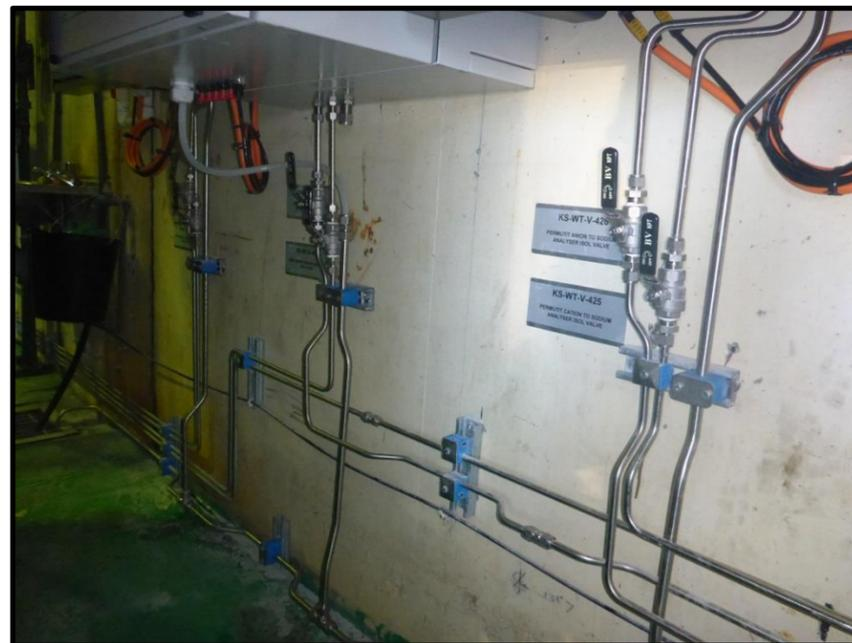
Figure 1: Analyser Tubing
