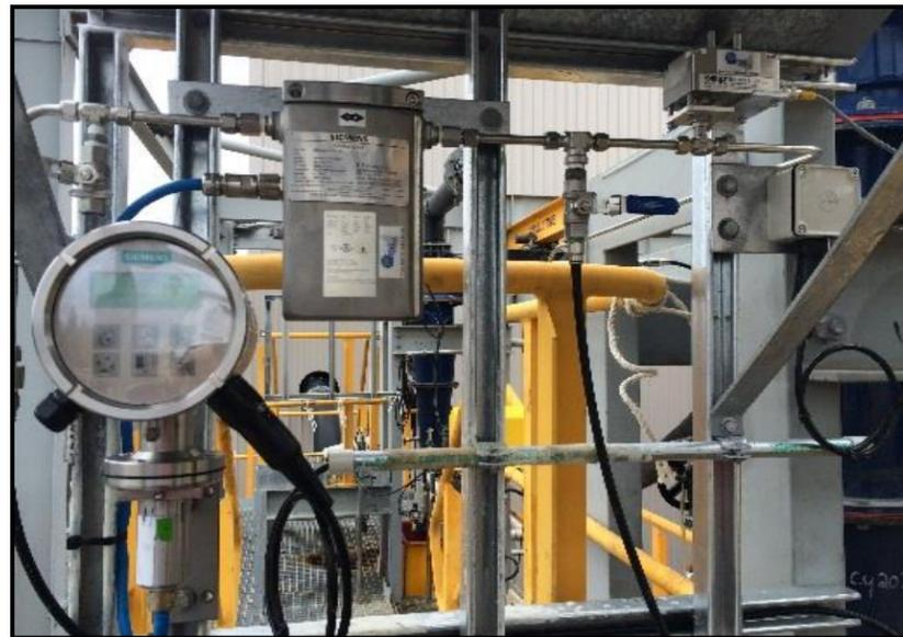
*The neat installation of the Siemens Coriolis flow tube, transmitter and the Hanbay actuator completed by the process plants own E/I department.*
