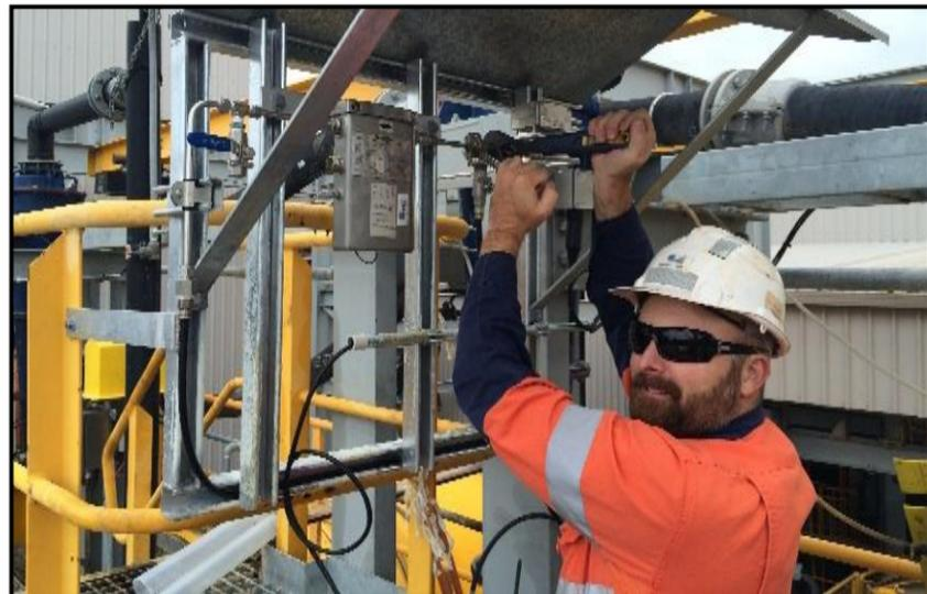
*Instrowest technician commissioning the new Hanbay actuator and Siemens Coriolis flowmeter*
