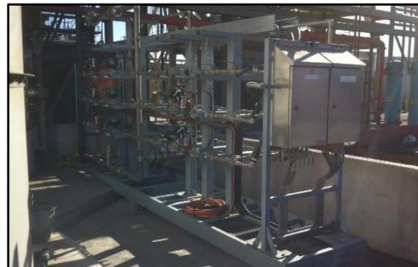
Full valve sizing was conducted by the Instrowest team; this enabled us to select the right size valve for the particular flow rate for each dosing line, V-Notch ball valves to give accurate control at both low ranges of flow and high ranges and being ball valves these also have the advantage of reduced chance of blockage as well as self-cleaning in their action.
